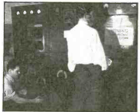
2—N.Y.A. junior workers adjusting controls of a 2,500-W. transmitter, sent to Quoddy Village by the C.A.A., soon to be modified for ham radio. The Quoddy N.Y.A. is now building the new Maine State Police radio system which is to comprise 2 headquarters stations and 15 mobile units; in the near future the system will include 6 headquarters points and about 95 mobile units.
